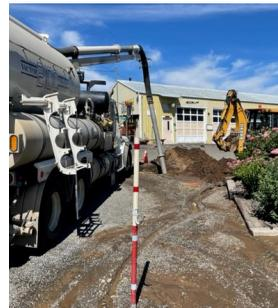
City of Union Gap crews working on repair of broken water main
