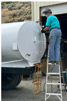
Bill Allen welding the valve at top of water truck
