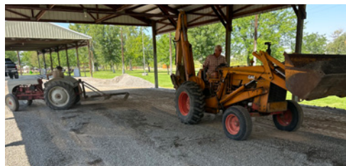
John Kobli spreading gravel in Building 18, while Kent Blomgren levels it
