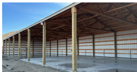
The new Stuart Gallion Building is 96 x 36 x 12 feet
