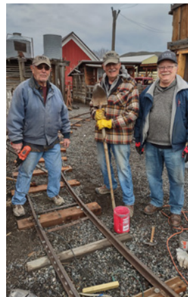
Harvey Cleem, Terry Stewart, and Greg Wilder working on the track
