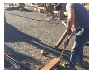
Matt Cleem pounding a new tie into the track for the kiddie train
